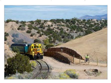
Vertical separation combined with a fence and retaining wall on the Santa Fe Trail in New Mexico. (Photo courtesy of Scott Belonger, P.E., Associate Principal for Loris and Associates)
