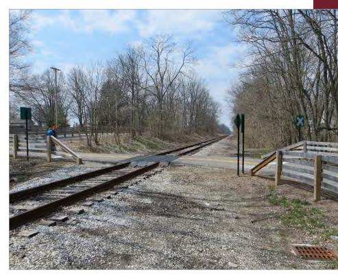
A trail/track crossing on the Camp Chase Trail in Ohio. The trail bends in order to cross the tracks at 90°. (Photo courtesy of the Rails-to-Trails Conservancy)
